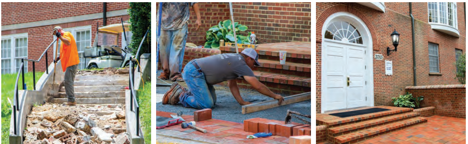
Rebuilding of the E. W. King Building brick steps and walkway
